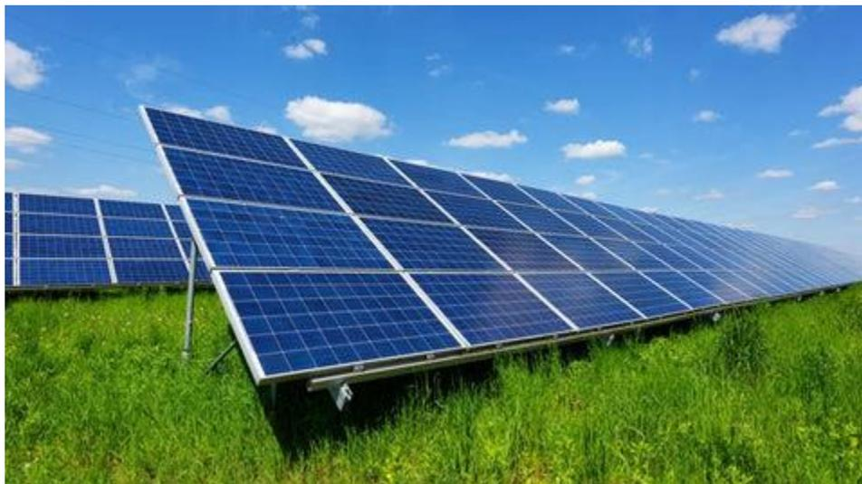
Solar panels use the photoelectric effect, also called the *photovoltaic effect*, to generate electricity from sunlight. When photons of light hit the solar panel, they knock electrons loose from the atoms in the solar panel. These electrons flow through the material to create an electric current. The more photons that hit the solar panel, the more electricity is produced.
